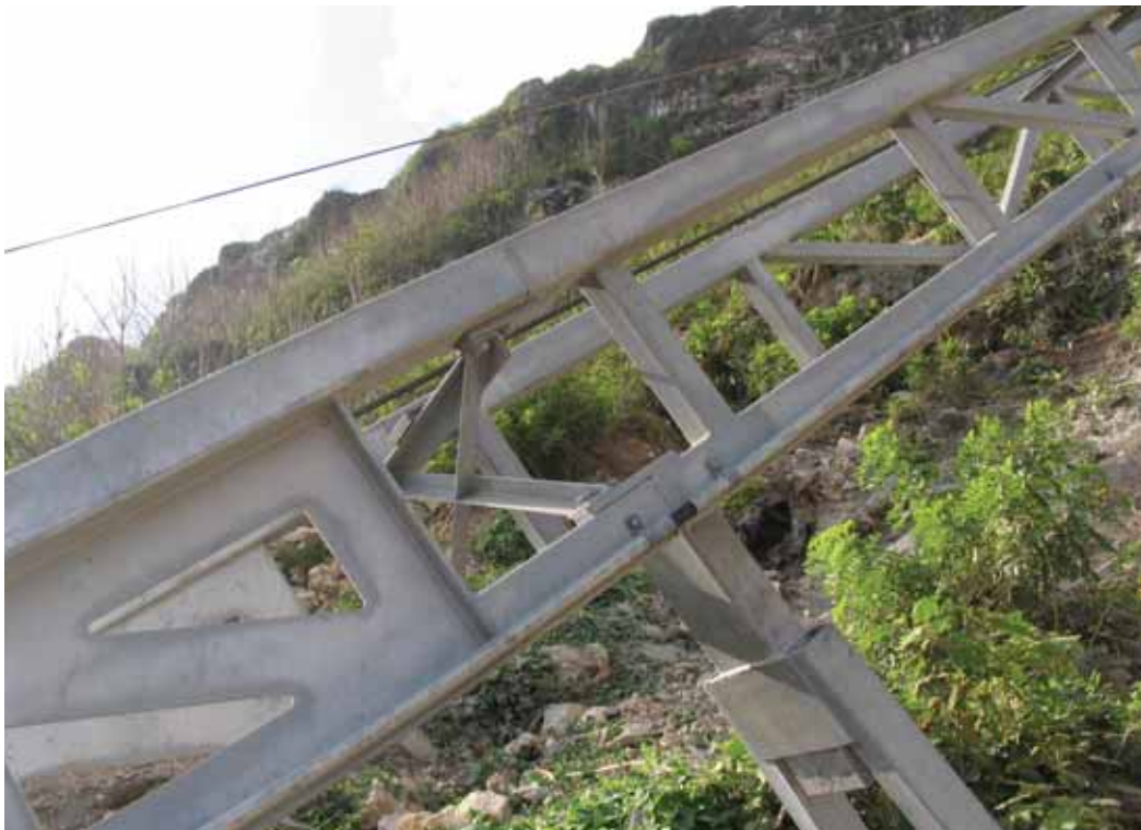
Top left: A sheave assembly and bogie cutout Top right: Detail of the cabs roof venting Bottom: A close-up of the rail structure
