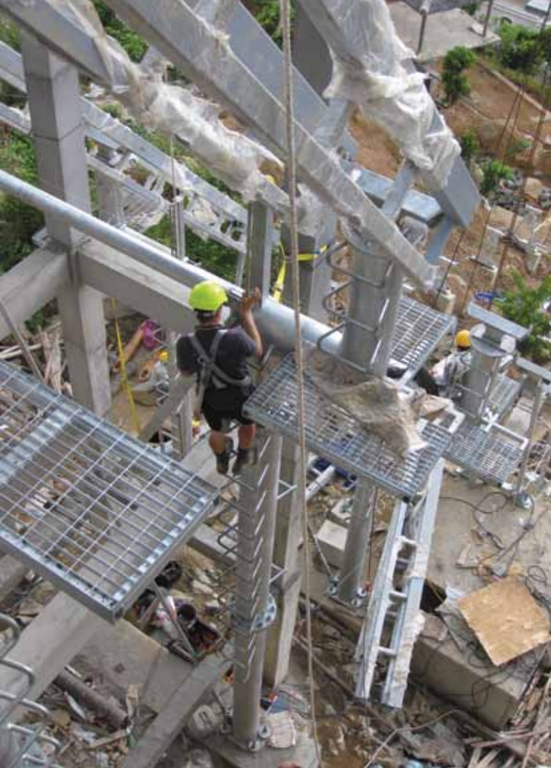
Construction of the foundation frames
