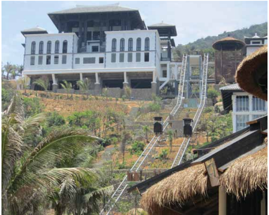
Nam Tram installations
